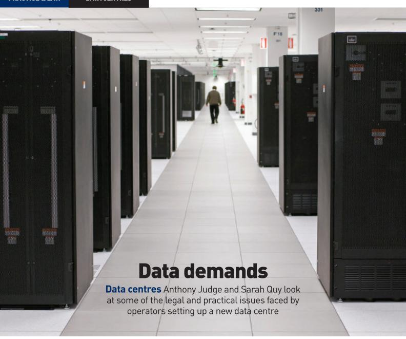
data centre is a space where companies locate and operate the ICT infrastructure that supports their businesses, including the servers and storage equipment that run software, and process and store data and content. This infrastructure can be a simple cage or rack of equipment, or a whole room housing several such racks. The facility will typically have a raised floor with cabling ducts underneath to power the cabinets and to carry the cables that connect the cabinets together.
